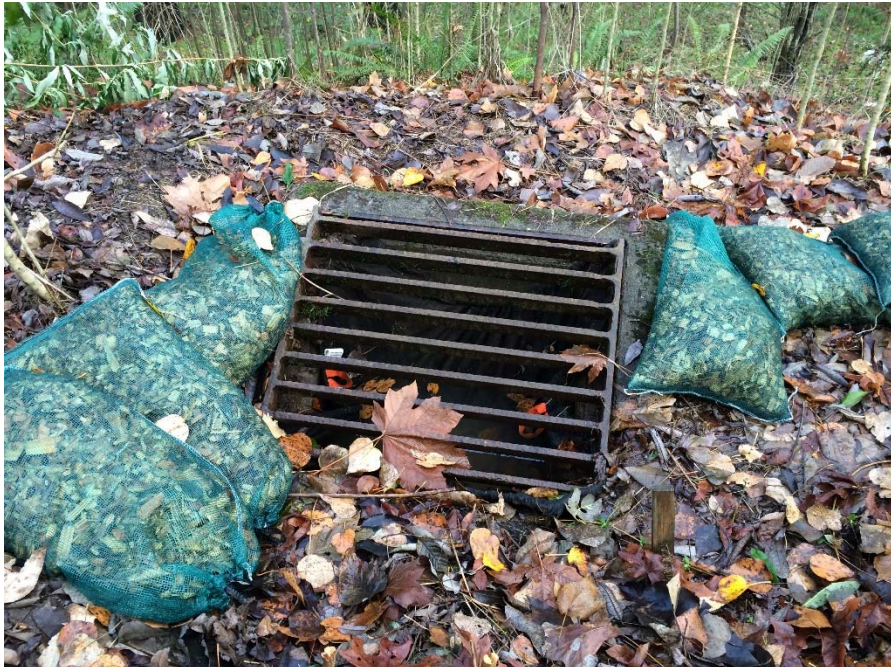
Photo 6: Catch Basin with wattles and stormwater inlet protection
